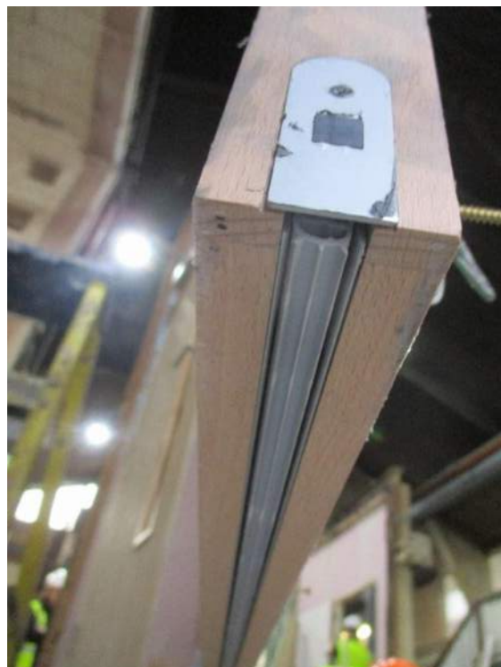
Figure 27 Drop down seal - Doorset A
