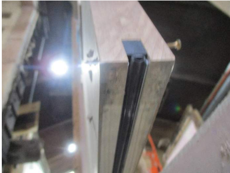
Figure 28 Drop down seal - Doorset B
