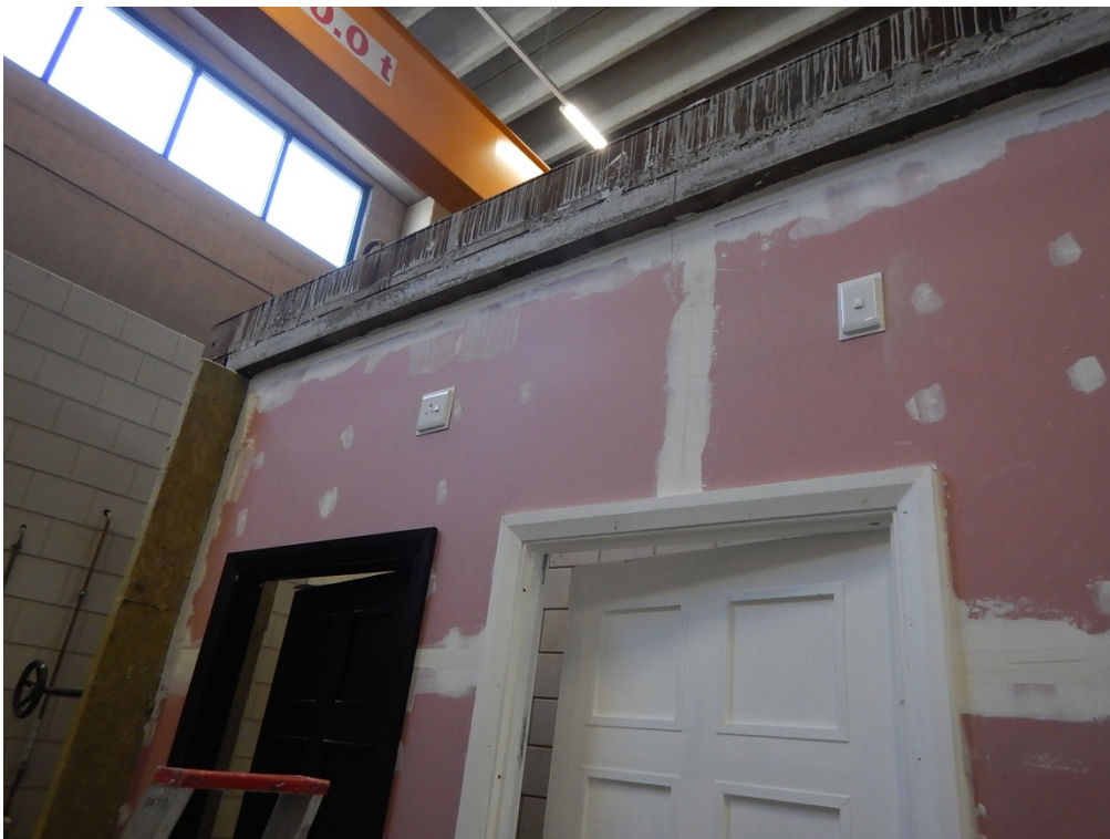
Foto C.8 Front view of the specimen after installation
