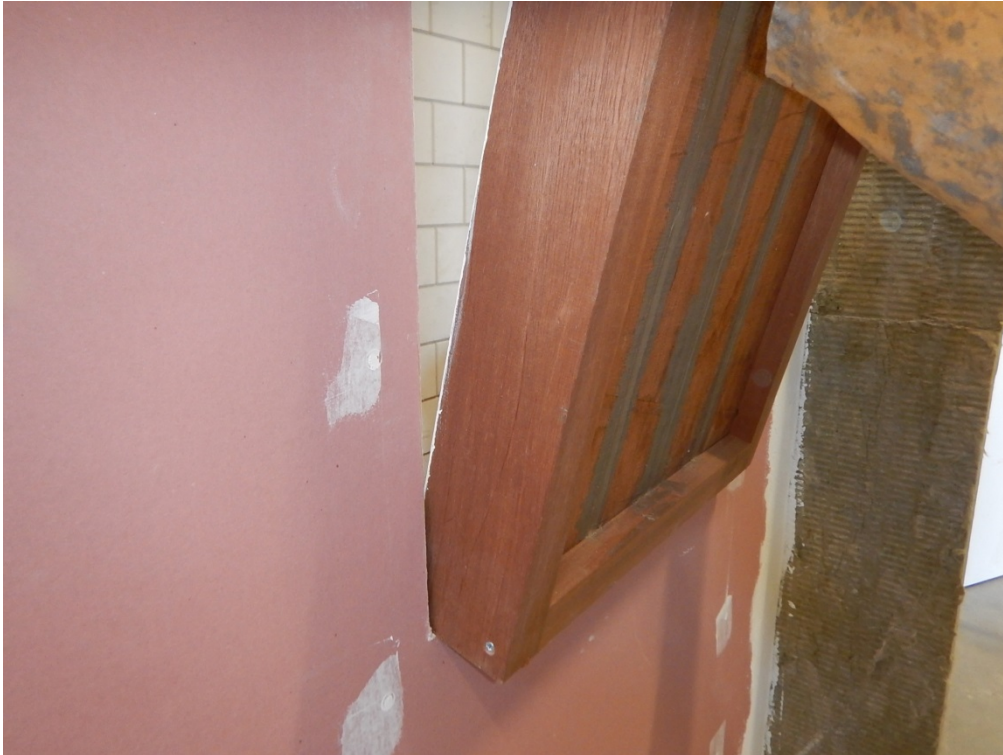
Foto C.3 Installation of the panel with the woodfiller product
