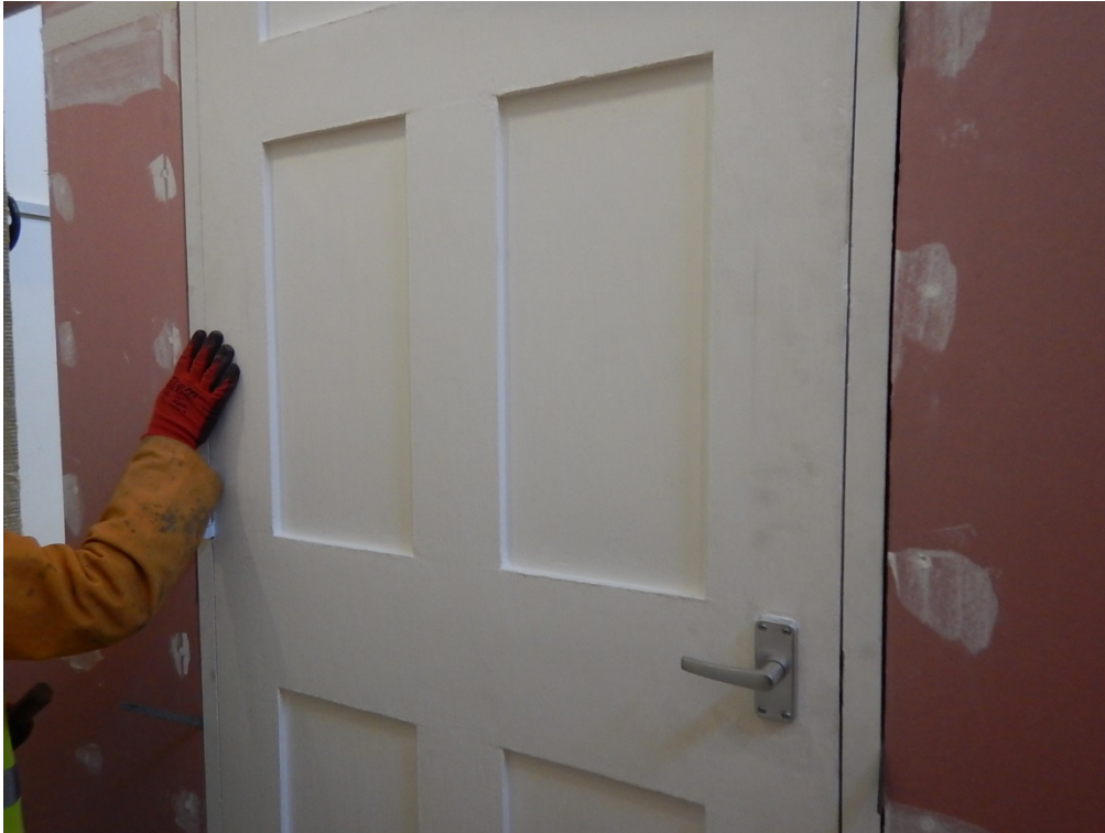
Foto C.1 Installation of the white door
