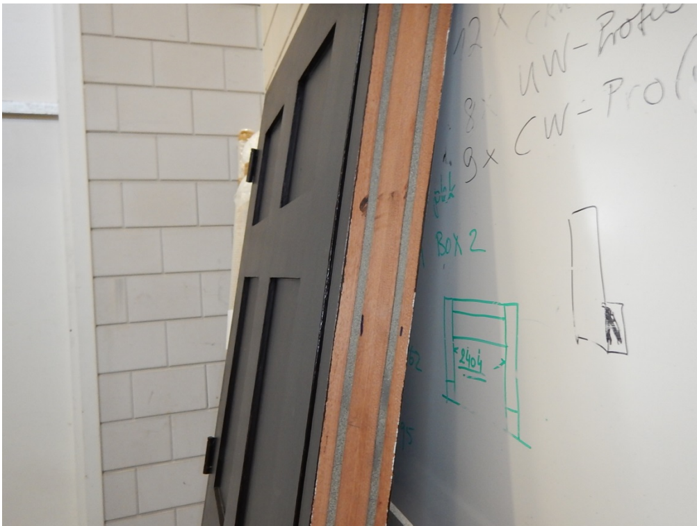
Foto C.2 Brown door before installation
